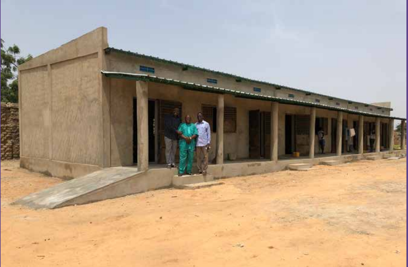
School of Hope Property During Construction
